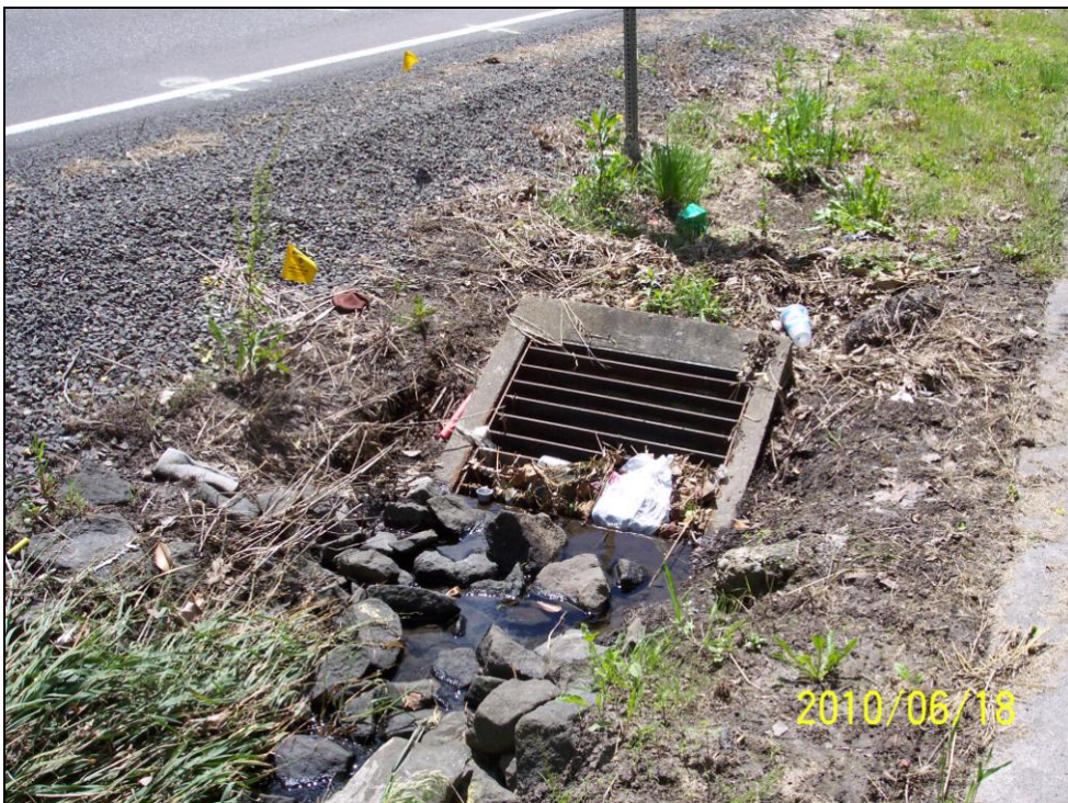
Photopoint 8: Rock lined roadside ditch terminates at culvert (taken 6/19/10)
