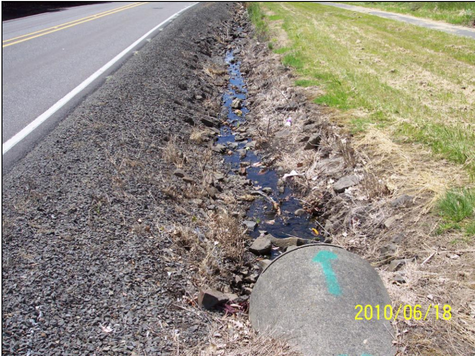
Photopoint 7: Rock lined roadside ditch with ephemeral flow (taken 6/19/10)
